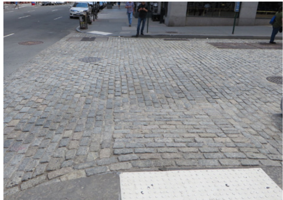
Figure 10: Harrison Street’s 2011 crosswalk reconstruction in Tribeca
