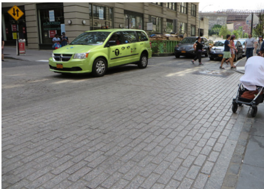
Figure 19: Phase One intersection with new thermal finish pavers at Front and Washington streets
