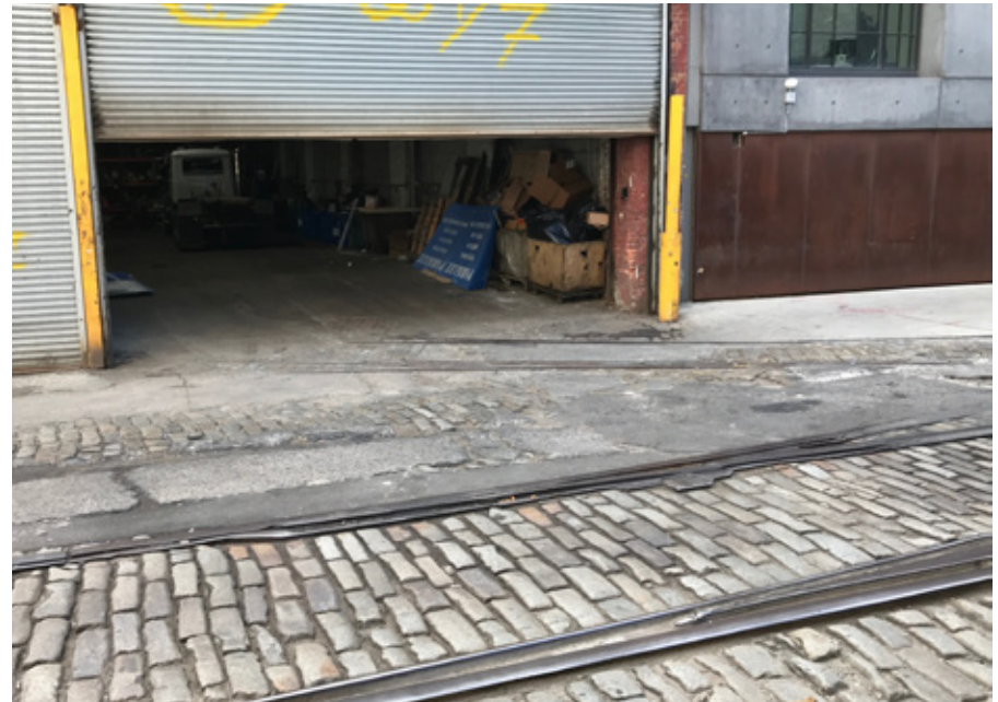
Figure 17: Rail tracks entering a building on Plymouth Street
