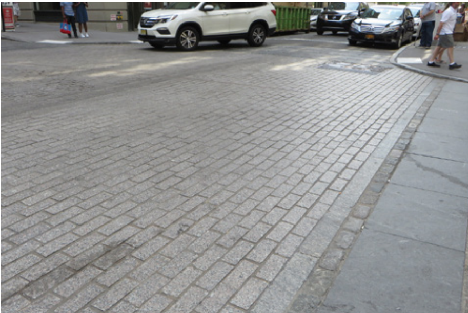
Figure 7: Front Street at Washington Street, showing new granite blocks installed within the interior of the intersection
