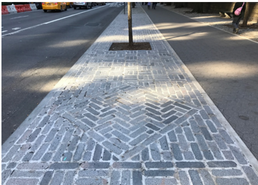
Figure 29: An adjacent bus stop with the Tumblestone pavers
