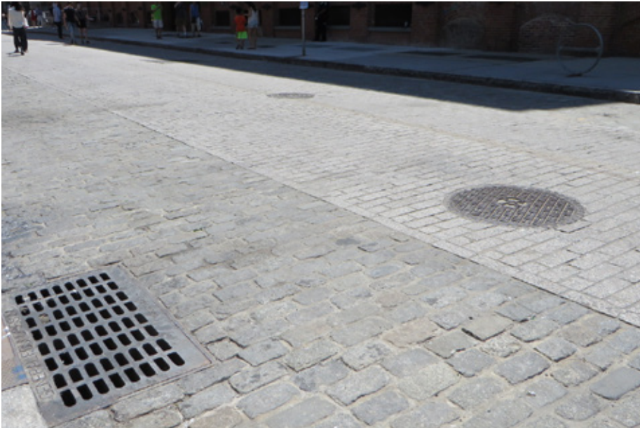
Figure 5: Washington Street's new center roadbed pavers (top) with historic Belgian block reset in the parking strip (foreground)
