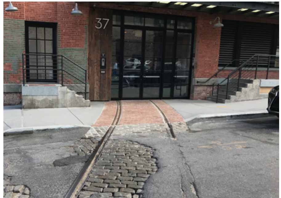
Figure 18: An attempt at ADA-compliant tracks at 37 Bridge Street
