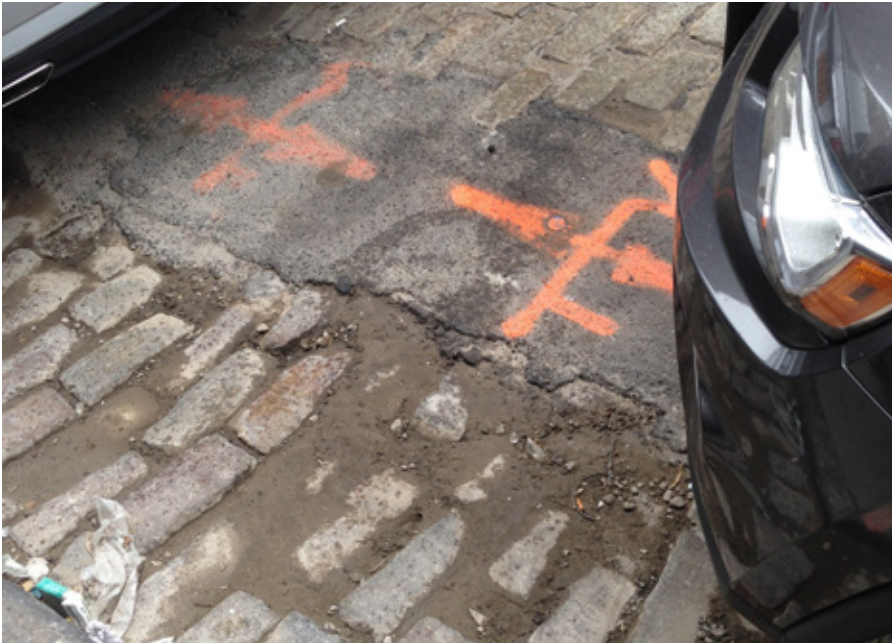
Figure 23: Asphalt patch and poorly reset Belgian blocks due to utility work in the roadbed
